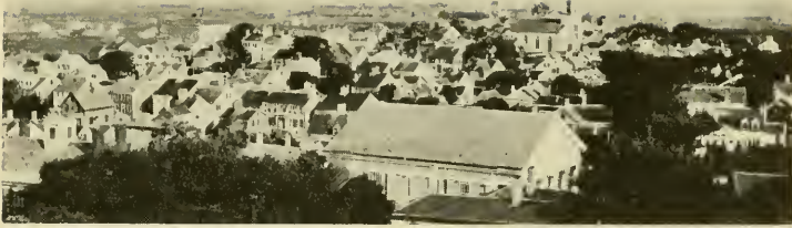
From the Tower Looking Toward the North Shore
